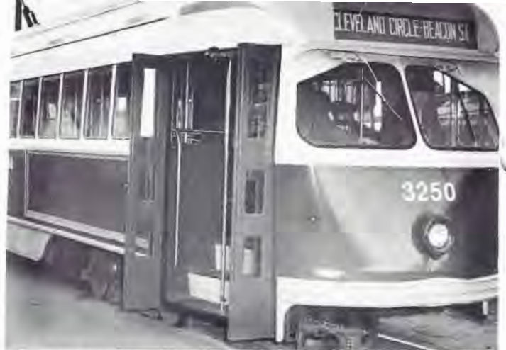
Eye appeal resulted when these two PCC's went through the MBTA's federally-aided program to refurbish 50 Green Line cars. Now, a directive has authorized the MBTA to rebuild 200 more PCC's over the next 2½ years. (MBTA)
